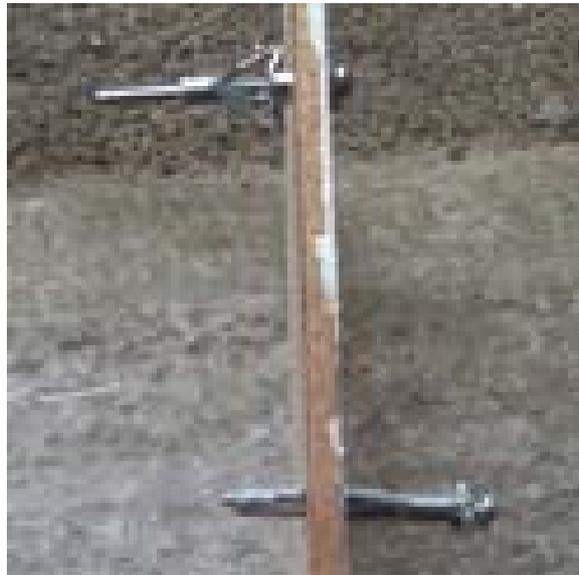
The hole is drilled in the board, an anchor pushed in. As the screw is turned it pulls up the body of the anchor. This grips the back of the plasterboard as you can see by the top picture.
